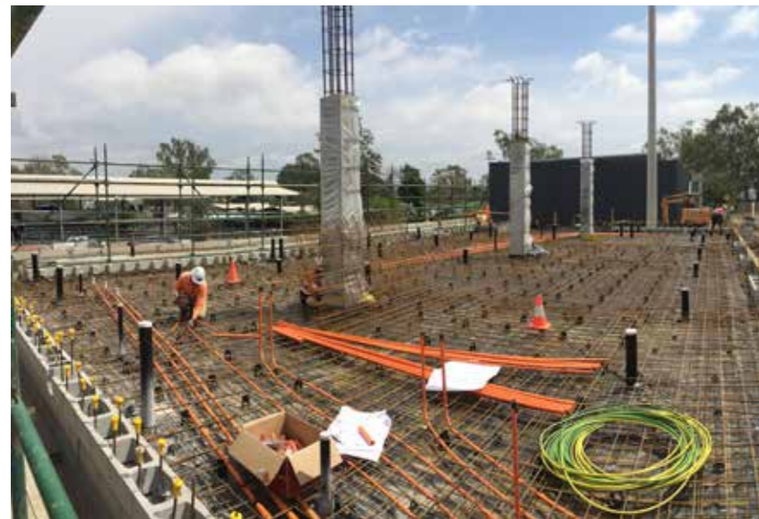
Construction of the new substation and chiller plant at UQ Gatton began during the year.
