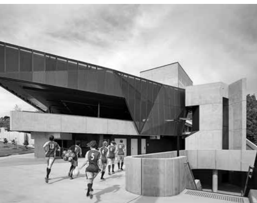
The remodeled Building 33, a central hub for athletes, supporters and function guests, overlooking the new synthetic sports fields for hockey and soccer, and constructed on a podium over a 500 car/350 bike-space covered carpark at UQ St Lucia. Photo: Christopher Frederick Jones.
