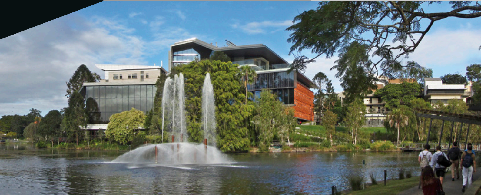
The Advanced Engineering Building opened in 2013 and was a collaborative project funded by the Australian Government, Queensland Government, and the University; with philanthropic support from GHD
