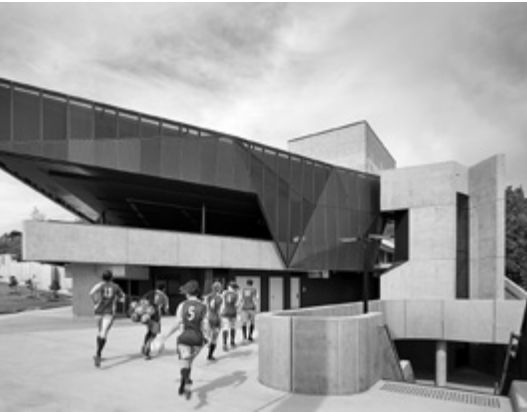
The remodelled Building 33, a central hub for athletes, supporters and function guests, overlooking the new synthetic sports fields for hockey and soccer, and constructed on a podium over a 500 car/350 bike-space covered carpark at UQ St Lucia. Photo: Christopher Frederick Jones.
