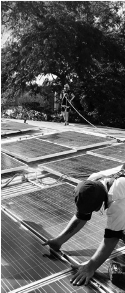
Installing solar panels at UQ's Pinjarra Hills site.
