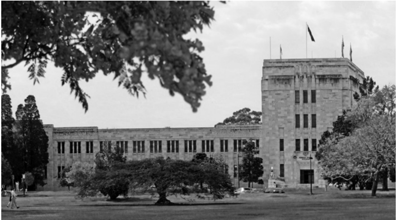
Levels 2, 3 and 4 of the Forgan Smith Building will undergo a major refurbishment in 2016.
